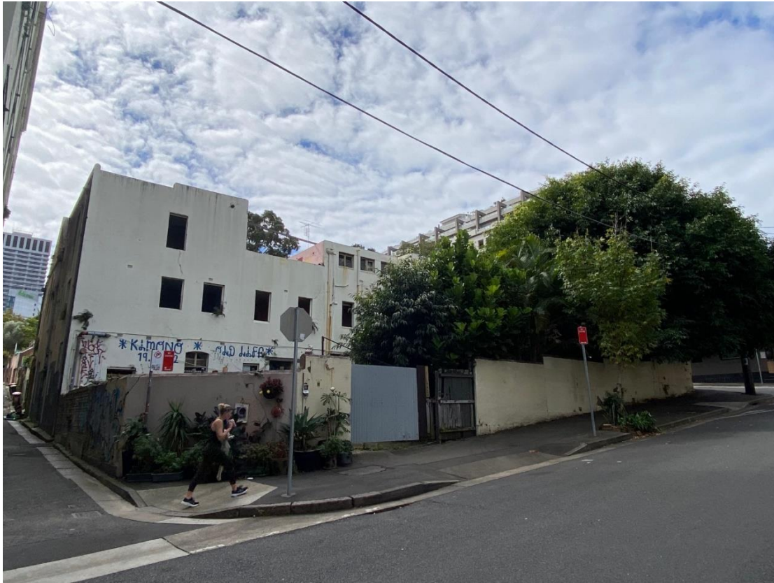
Figure 4: Site viewed from Reservoir Street, looking north-east
