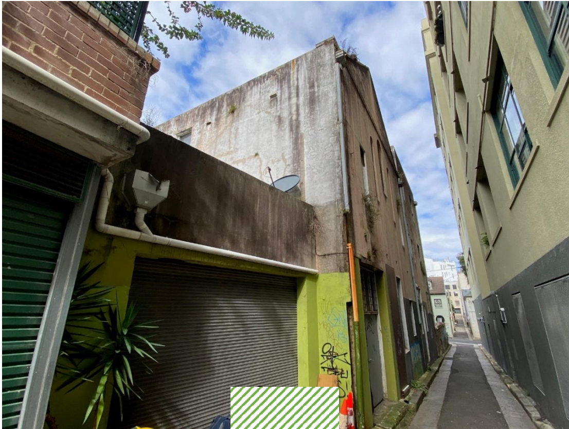
Figure 6: Site viewed from Beauchamp Lane looking south-east
