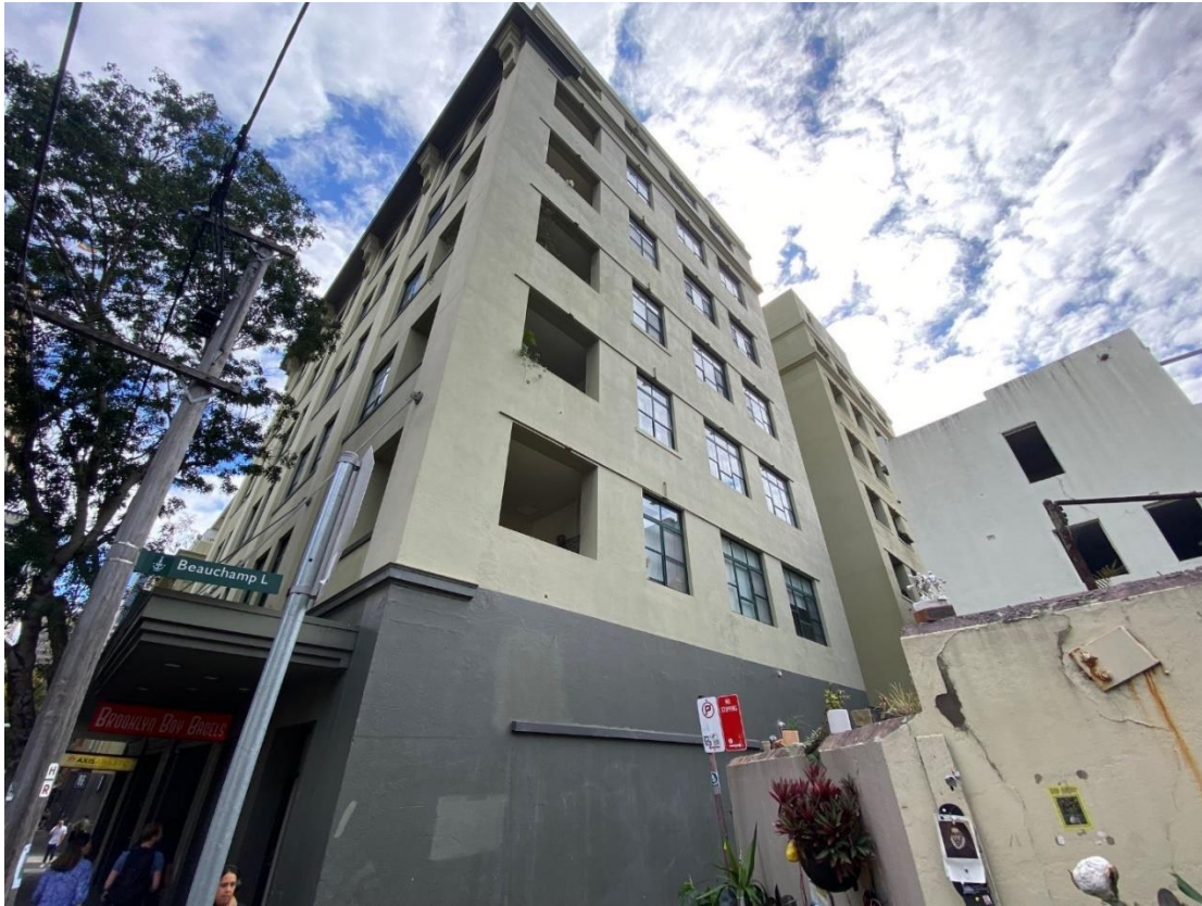
Figure 8: Neighbouring site to the west, viewed from Reservoir Street looking north-west
