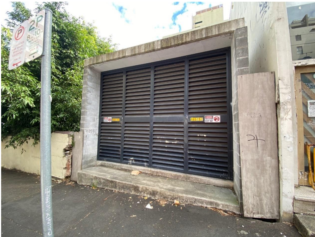
Figure 3: Existing substation proposed to be retained on Commonwealth Street frontage
