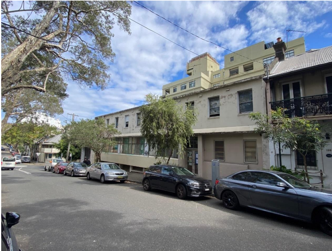
Figure 2: Site viewed from Commonwealth Street, looking south-west
