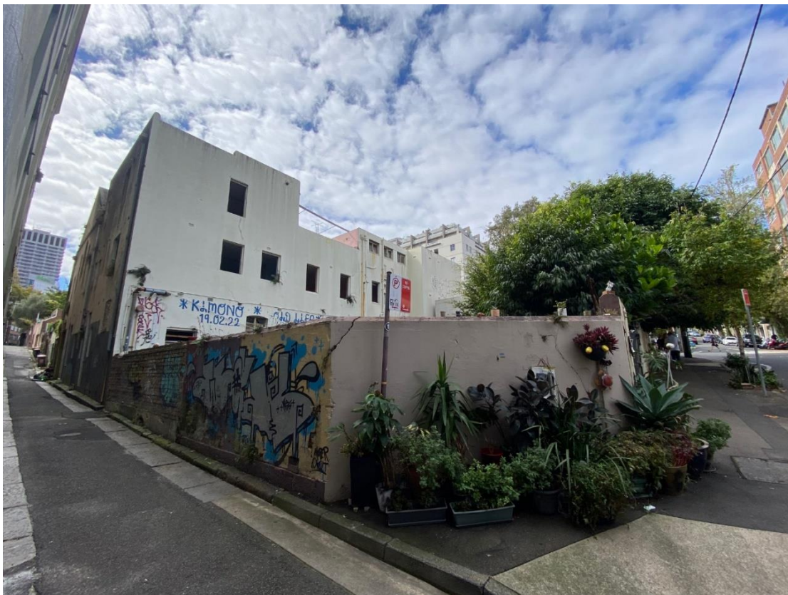
Figure 5: Site viewed from Beauchamp Lane, looking north-east
