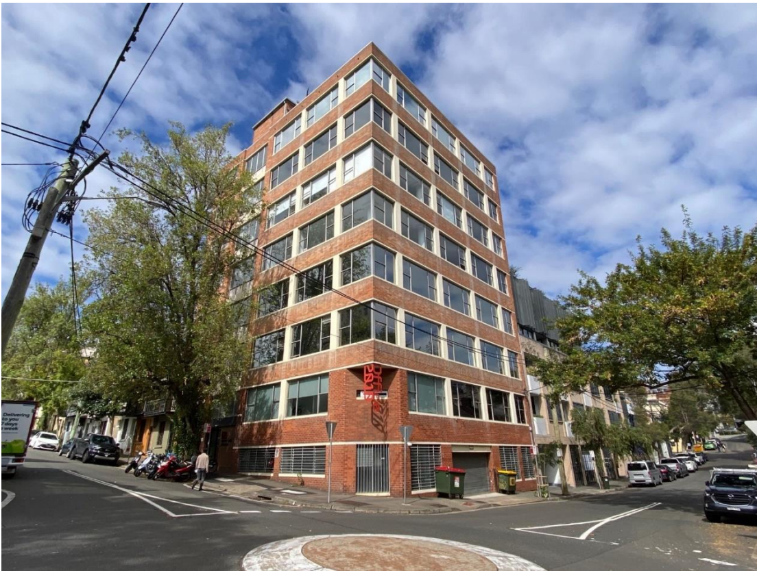
Figure 11: Existing development on Reservoir Street diagonally opposite to the south-east
