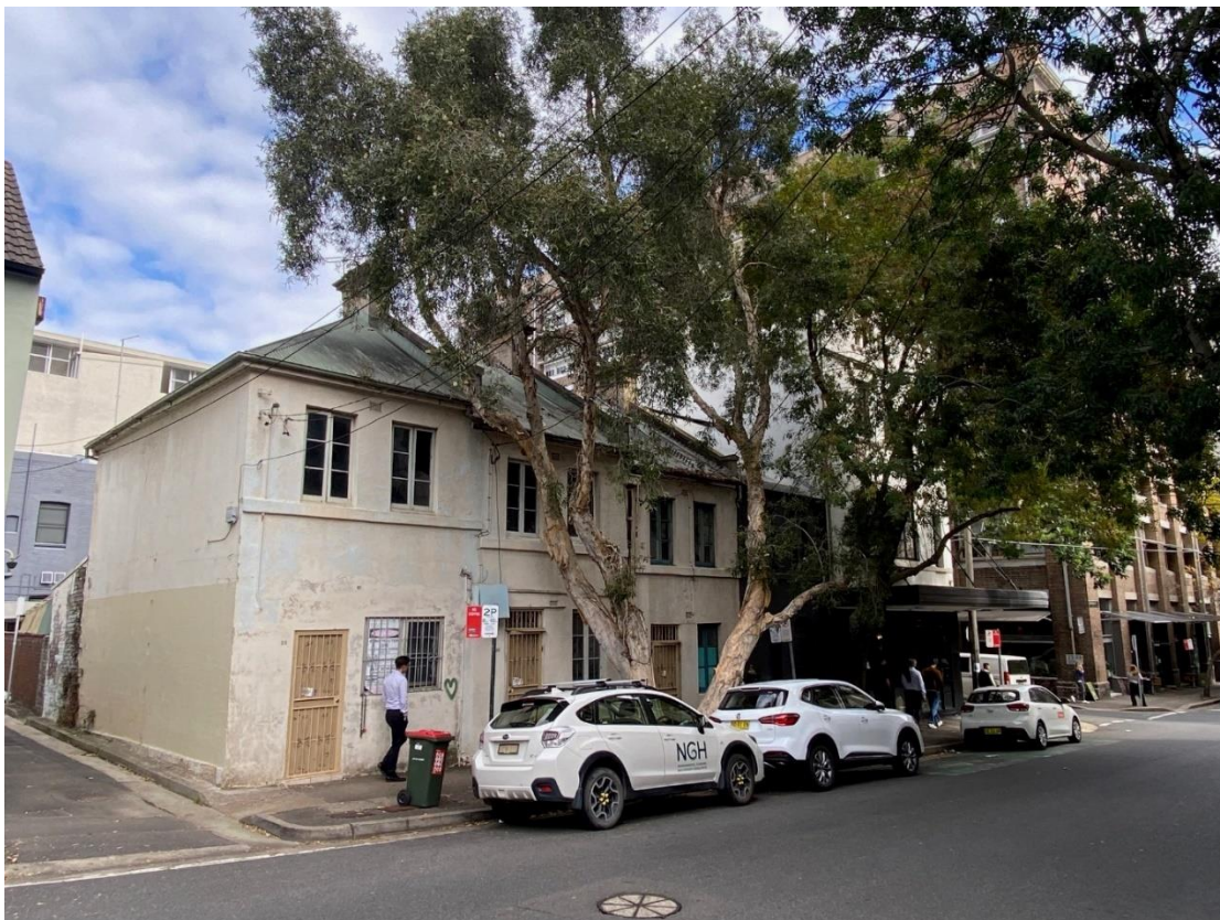
Figure 9: Existing development on Reservoir Street diagonally opposite to the south-west
